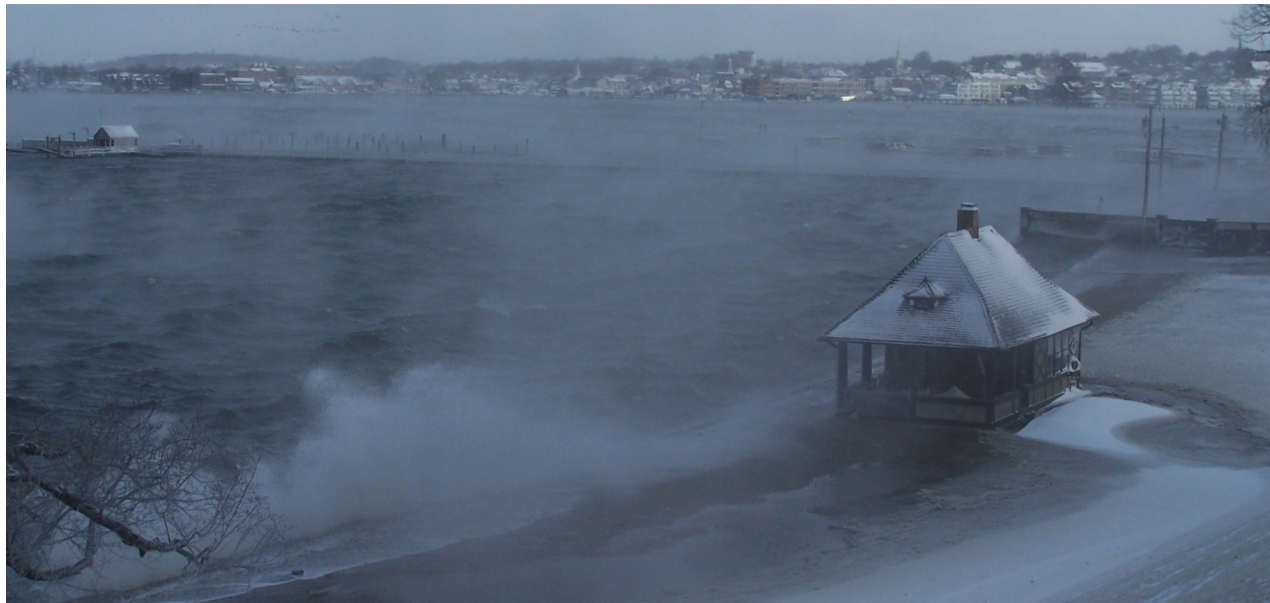
Seawater has been overtopping the seawall more frequently in recent years during storms and high-water events; the boathouse, a whimsical early 1900s structure, is also inundated regularly and needs to be moved slightly inland for protection.
